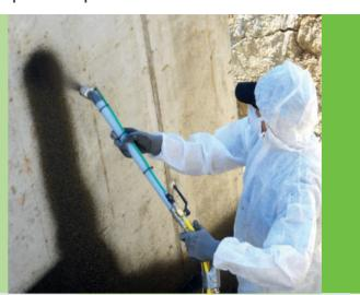
The **inoBEAM M8** delivery pump handles materials based on the "walk principle". A flexible rubber disc pushes the material to be conveyed through the pump housing and into the material hose. This delivers a considerable benefit: less frictional heat is generated and the material is conveyed very efficiently.
